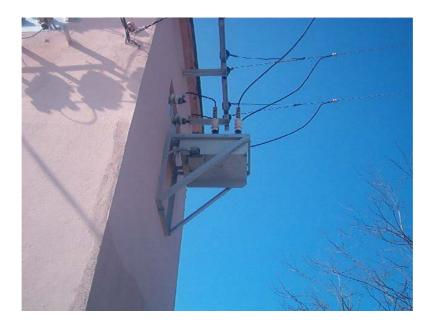
An RS485 RTU interface offering 300-19200 baud, full and half duplex modes is provided to connect to remote control systems. DNP3 protocol is provided in the standard combined which is incorporated in existing remote control system. Radio or modem can be used for data transfer. Concrete, the substation 'Samaila 1' used radio for data transfer.
