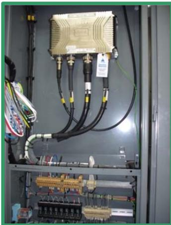
**Figure 3: PIU mounted in 11 kV switchgear**
