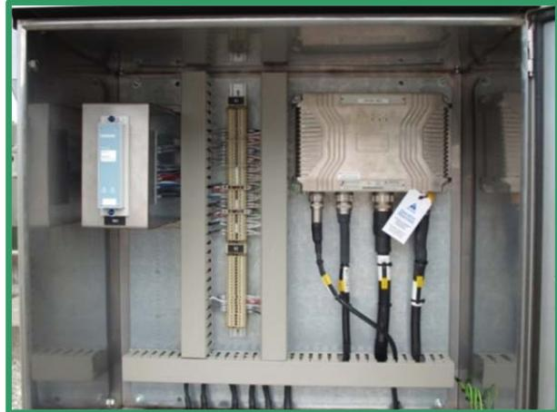
**Figure 4: PIU mounted in 33 kV breaker**
