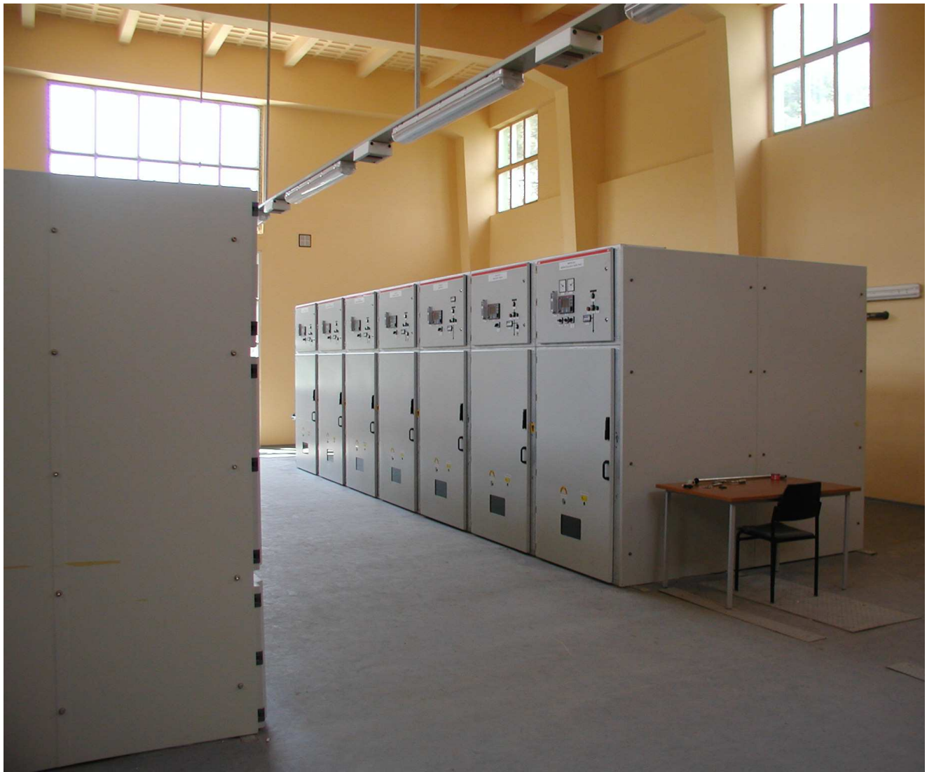
Figure 4 - Metal clad switchgear after reconstruction
