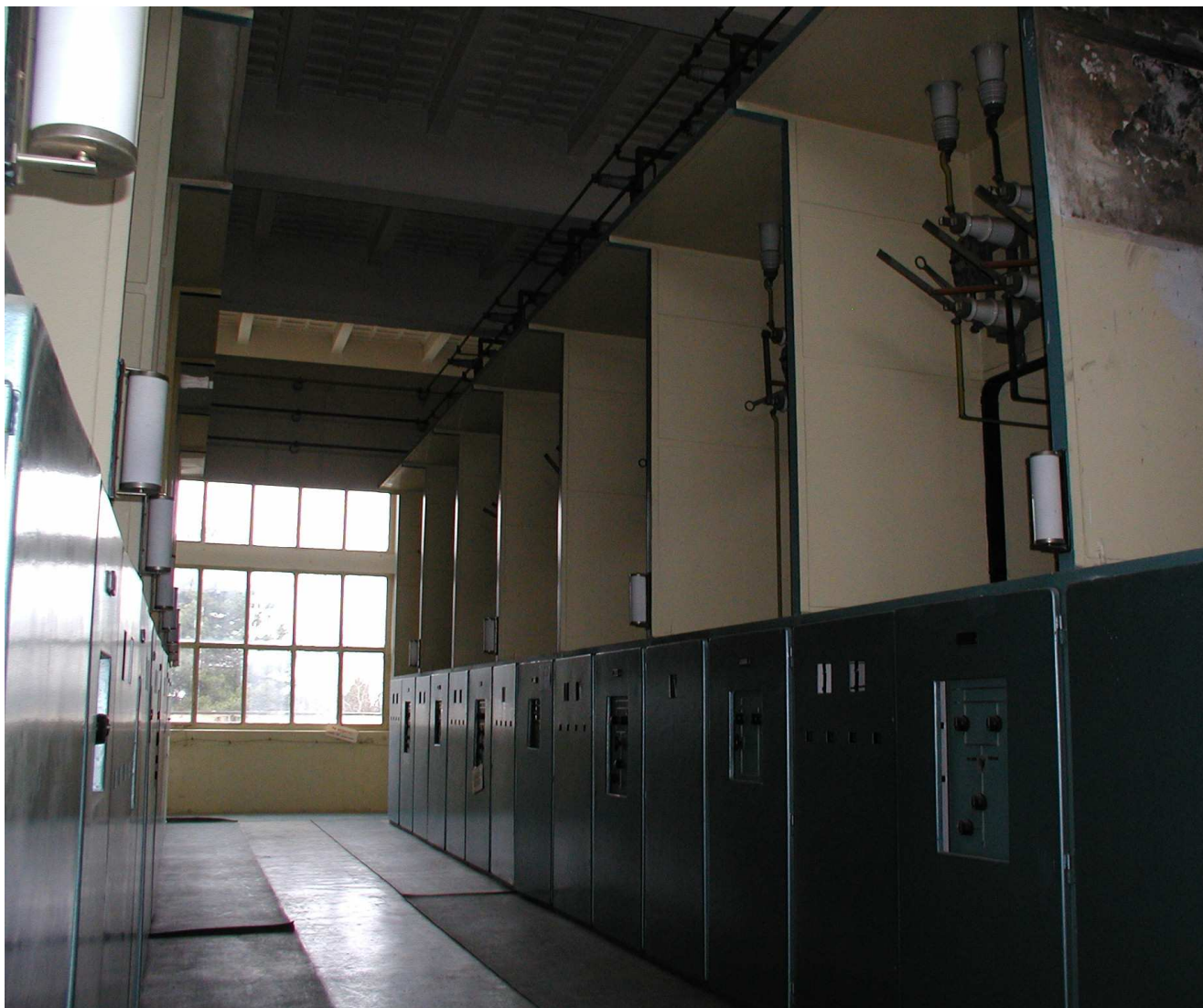
Figure 3 - Switchgear 35 kV before reconstruction
