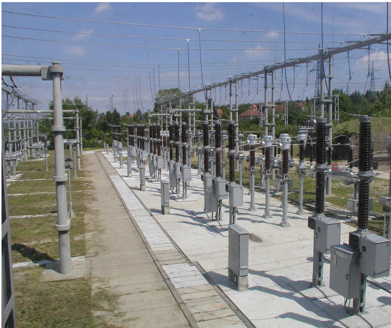
Figure 2 - Switchyard 110 kV after reconstruction
