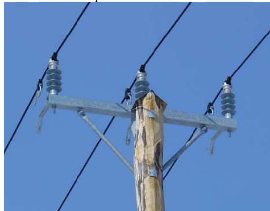
Figure 3: Example of overhead power line with composite insulators
