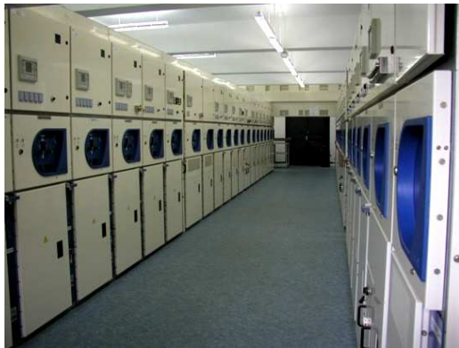
Figure 6. 6 kV bays in a modernized substation
